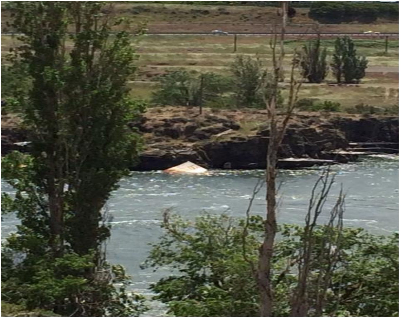
Failed tribal platform along Oregon shoreline across from Westrick Park.
